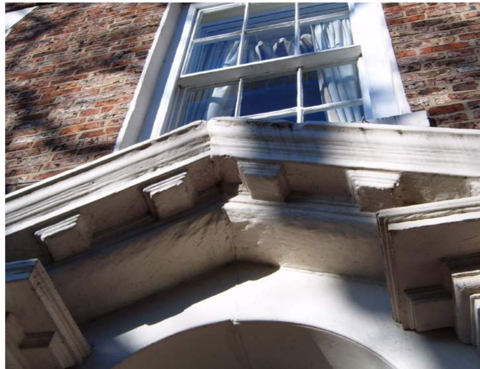
DETAILED VIEW OF THE MAIN ENTRANCE PORTICO
